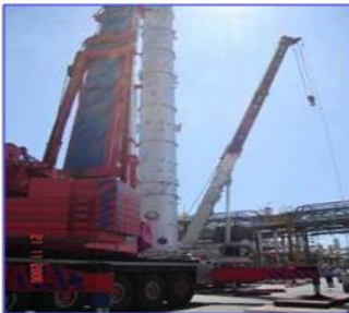
Size : 15,000 mm x 20,000 (AISI 316) Installation of Stabilizer Column
