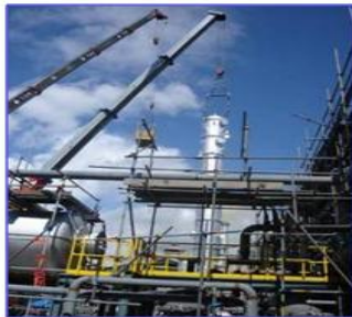
Size : 15,000 mm x 20,000 (AISI 316) Installation of Stabilizer Column
