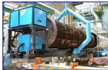
Complete On-Site Re-Tubing
