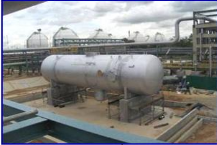
Size: \Phi 3,000 mm x L 13,000 mm Hopper
